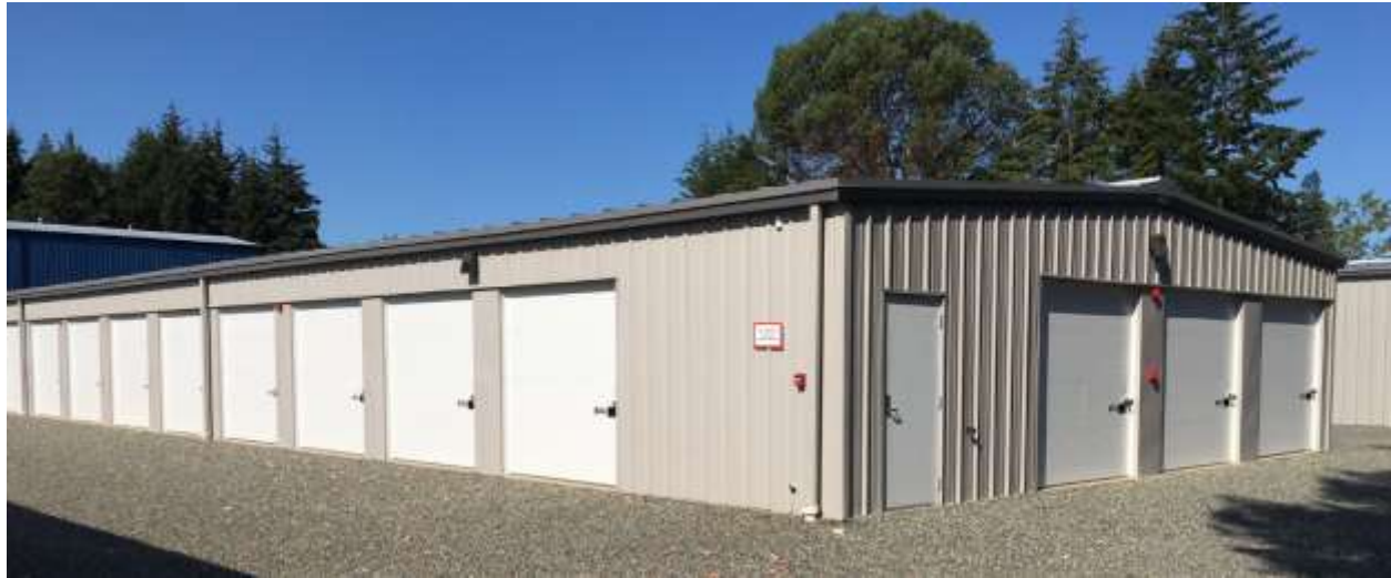
Figure 4: An Existing Mini-Storage Warehouse Building as an Example
